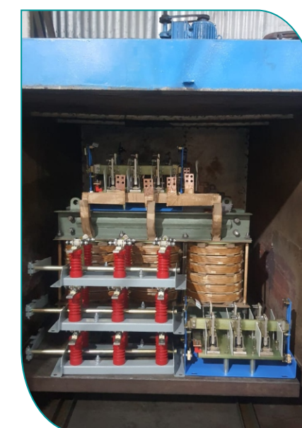
DTR'S PLACED IN BAKING OVEN WITH HV ISOLATOR & LV CFS
